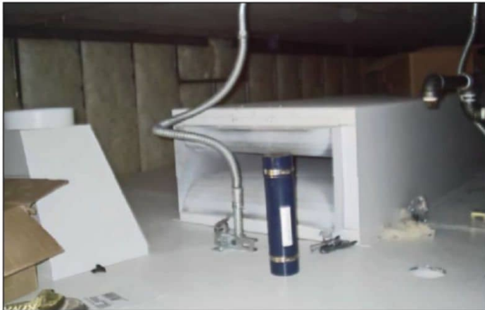
Photo 4: Sprinkler in the form of a duct. Coordination is important! The return air (RA) silencer and a conduit to a chamber light is shown here, this would have been quite interesting if it was the supply air (SA) silencer. (Image source: MSAI)
