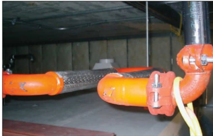
Photo 5: Sprinkler vibration isolation. Many chambers require sprinklers. Note the flex connections to the chamber roof mounted sprinklers. The yellow rope was removed when the construction was done. (Image source: MSAI)
