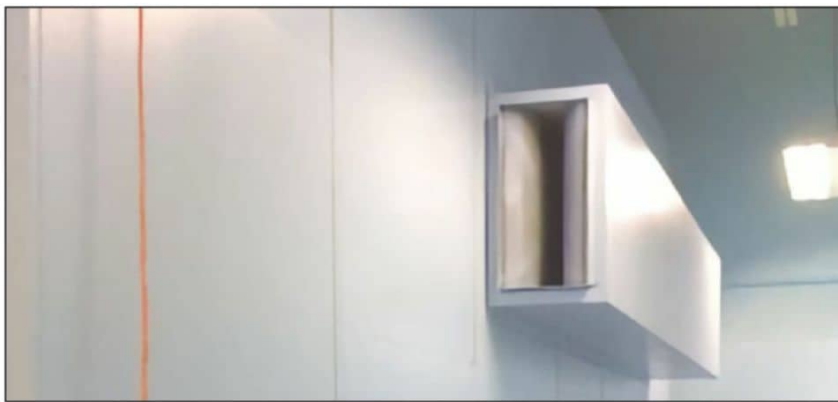
Photo 3: HVAC side silencer. We always need to remember the HVAC! (Image source: Eckel)
