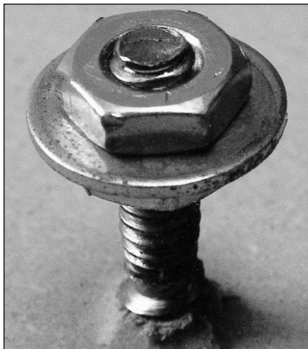
PHOTO 31: Mounting a hanger bolt.
